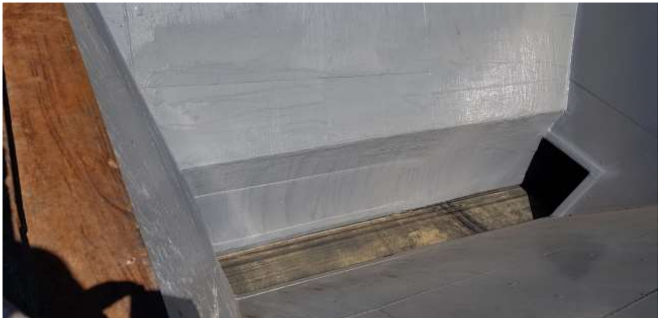
Manufacture of Wall and tunnel with MTS in the hopper.
