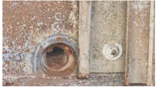
Inside of Cooling Tower, corrosion detail.
