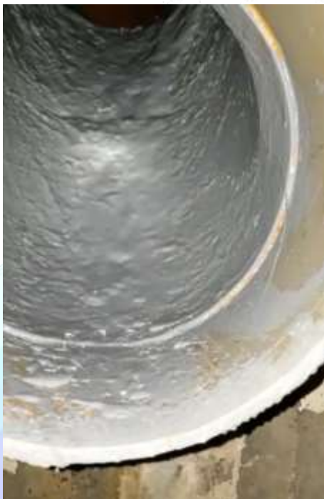
Downpipe elbow repaired with (MTS)
