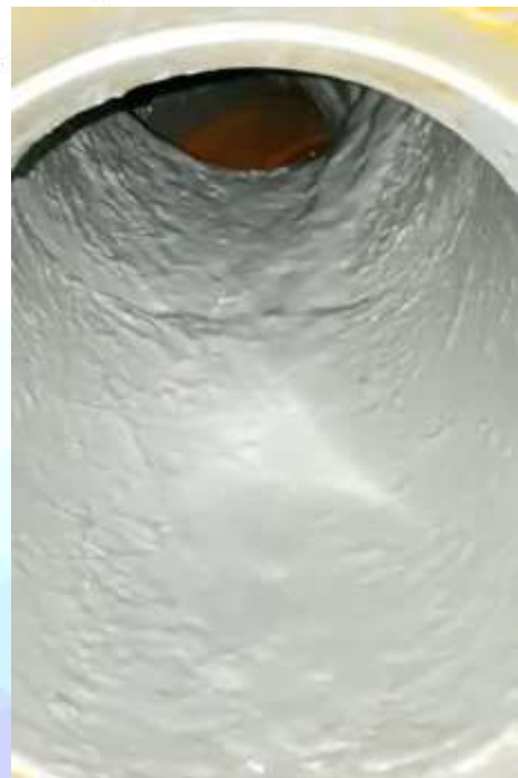
Downpipe elbow repaired with (MTS)
