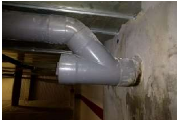
Initial state of downpipe elbow with the break.
