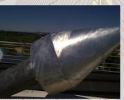
The surface required, as proper treatment, an exhaustive sanding to show a significant white corrosion of the galvanization as nitrate and oxide.
