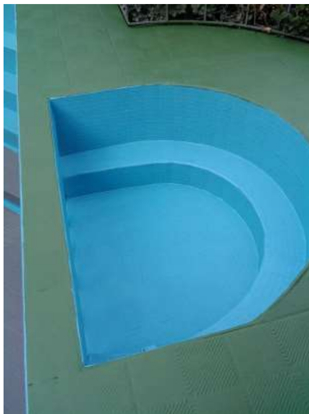
Vessel manufactures with MTS
