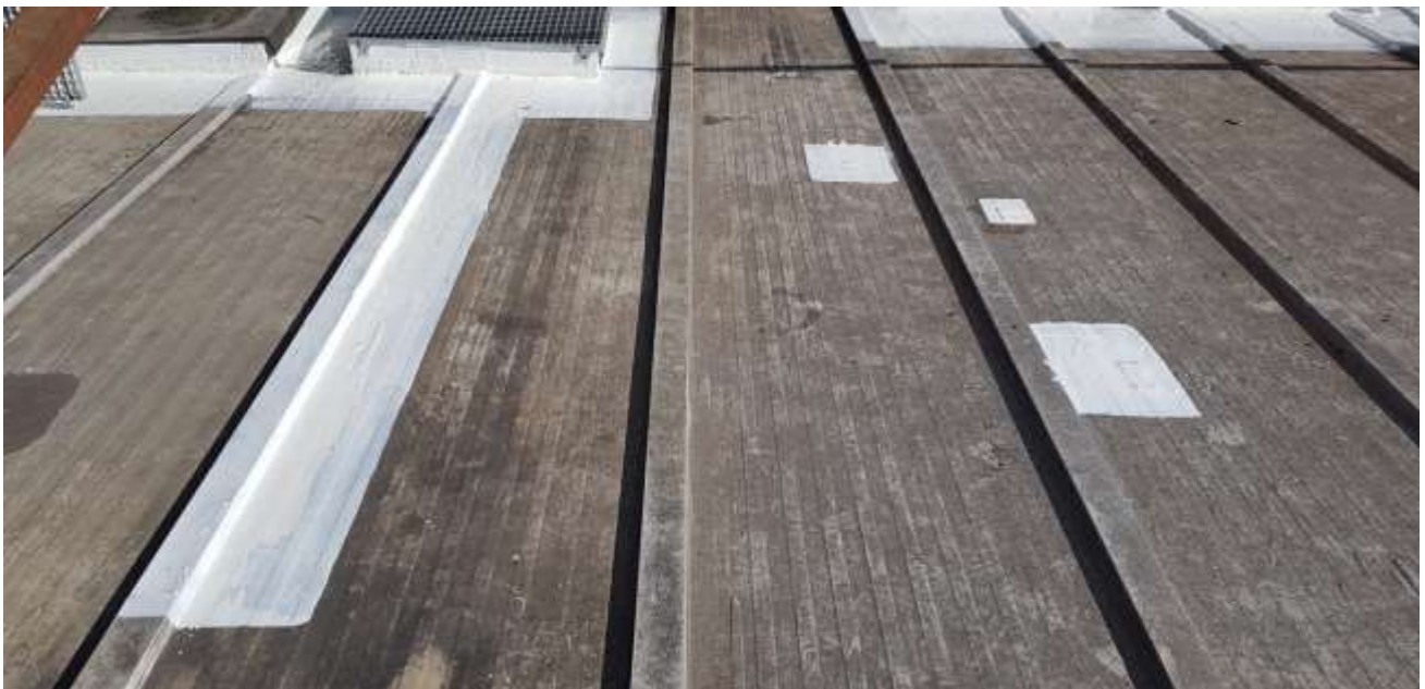
Detail of skylights and several zones of the roof waterproofed.
