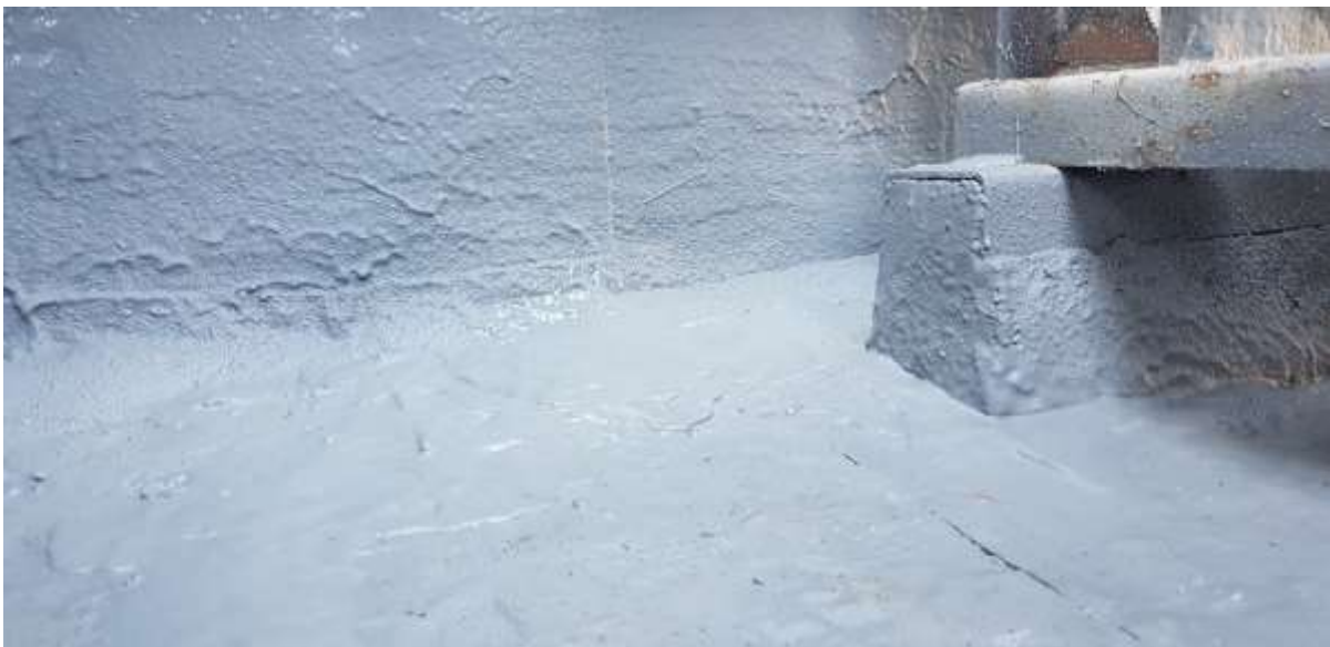
New roof manufacture with MTS.
