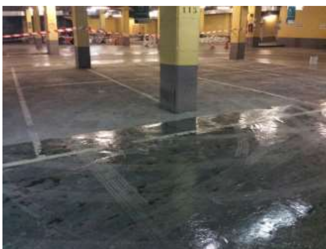
Cleaning, sanding and surface preparation
